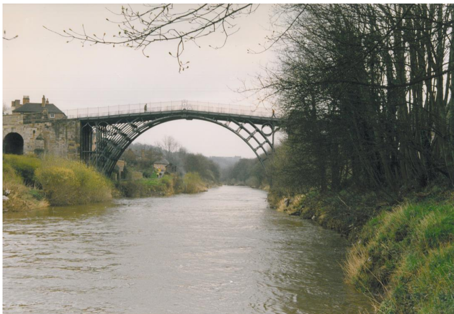
1. ábra. The Iron Bridge over river Severn. Toll Bridge. Épült 1779 (Coalbrookdale, UK World Heritage Site (Courtesy of Gordon Clark)
